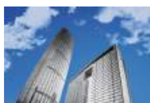
In-Building - PABX Integration
